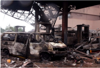
Kwame Nkrumah Circle gas explosion (Twin disaster) in 2015
