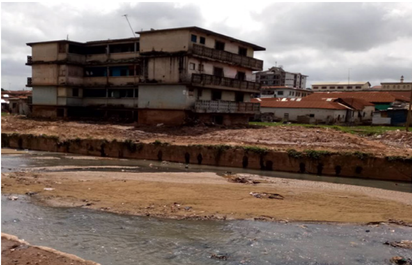
Figure 5.1: Disaster-prone settlement at Aboabo in the Ashanti Region of Ghana.
